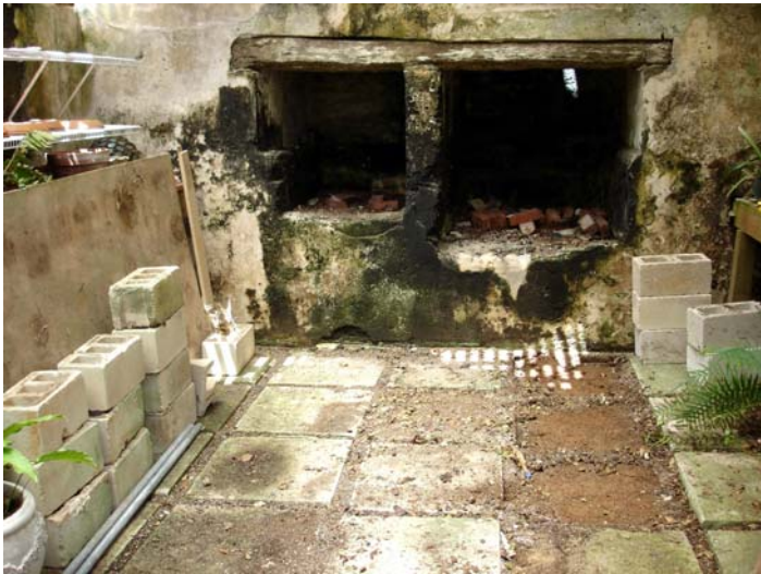
Figure 15 View of out-kitchen fireplace in slathouse. Note the bake oven, cooking fireplace and single step bench.
