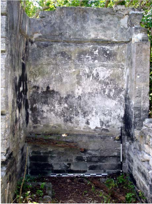
Figure 28 Photograph of closet E in Hallway F.
