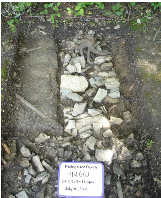
Figure 65 North wall foundation (bottom) and perpendicular wall of the vestibule.
