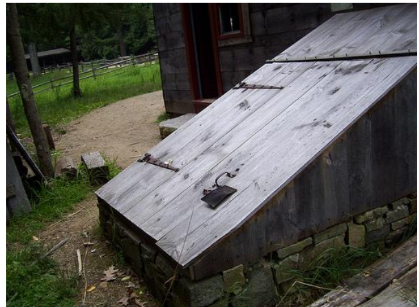
Figure 71 Bulkhead style cellar door such as may have been on the west side of the Presbyterian Church based on features found in N1W14.
