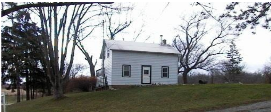
Figure 55 Hill House, ca. late 1830s/early 1840s (Stokes 1995) in Ruthven Park N.H.S., is considered to be the only surviving example of Grand River Navigation Canal Co. tenant housing.
