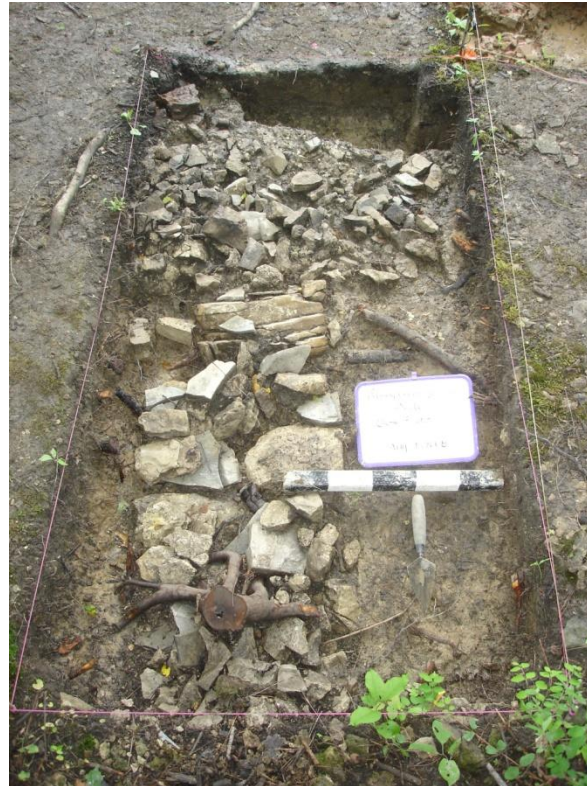
Figure 77 View looking south showing the narthex/vestibule foundation running north-south and the building foundation running east-west in the background. The different size stones indicate different phases of construction. The edge of the cellar pit was discovered on the inside of the foundation wall and is shown partially excavated here (upper).
