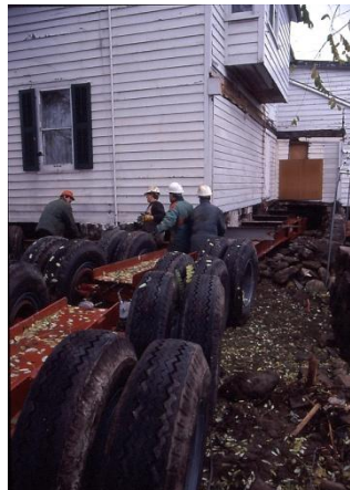
Figure 35 Modern house moving employs similar technology as that used during the 19 th century – jacks, temporary frames and wheels.
