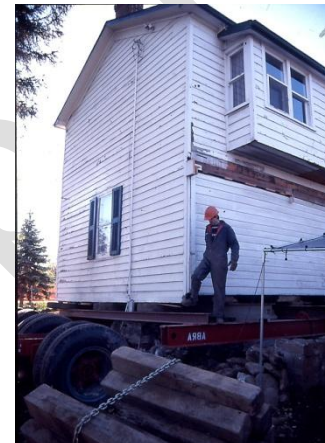
Figure 35 Modern house moving employs similar technology as that used during the 19 th century – jacks, temporary frames and wheels.
