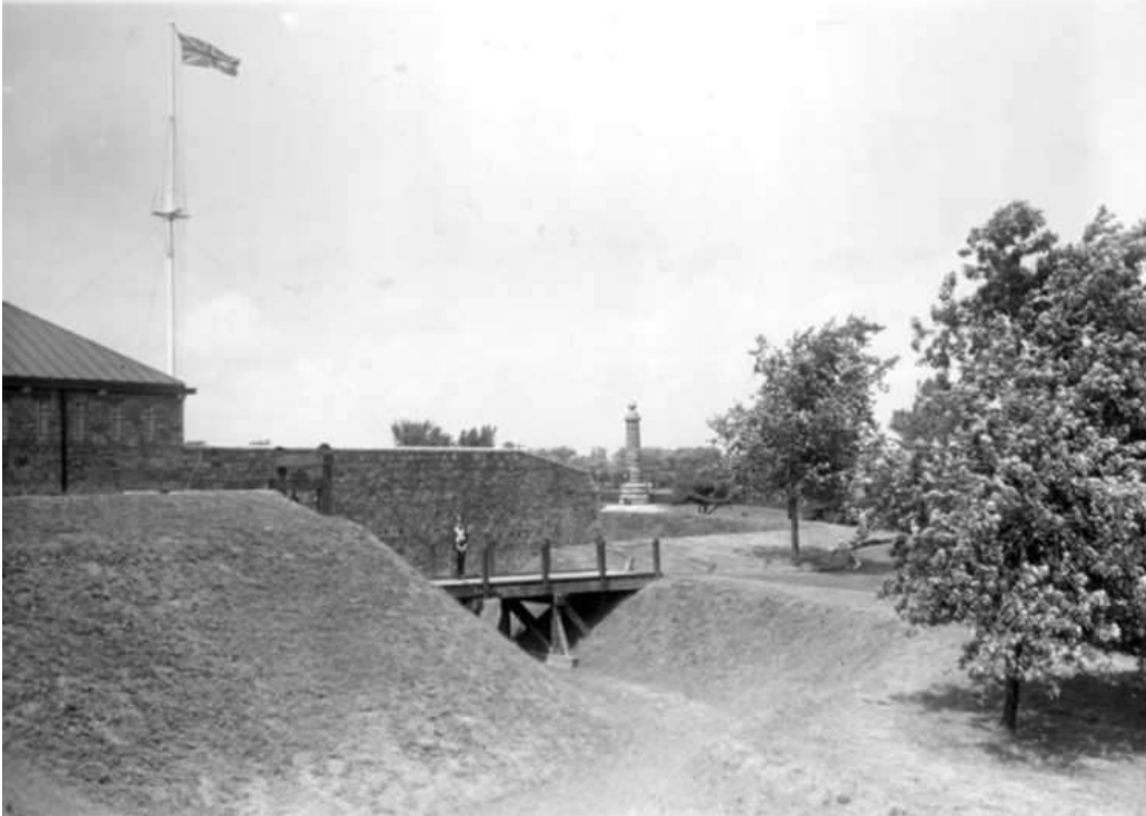
Figure 21 The Old Fort Erie – 1939, Francis J. Petrie Collection, July 30, 1939, after restoration. Niagara Falls Public Library Digital Collections, Record ID 94943. Photo probably taken from atop Douglass Battery. (2013 excavation area to right of photo.)
