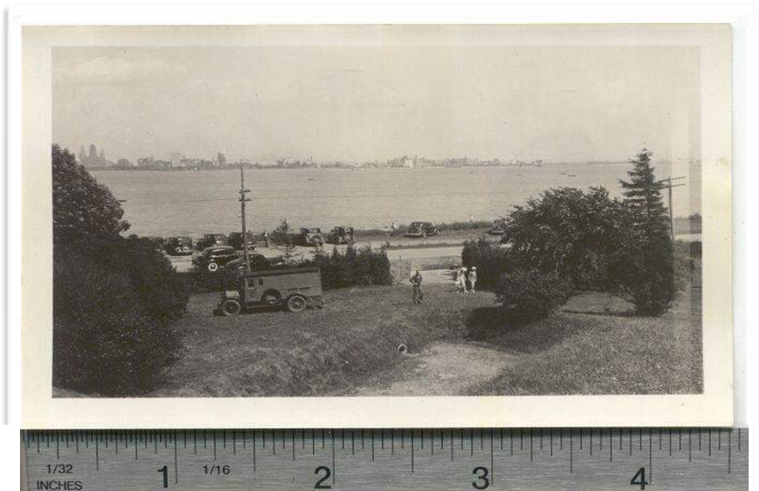
Figure 30 Photograph dated 1939 showing lakeside entrance to fort. The drain found in Unit B can be seen in the mid-foreground draining the ditch surrounding the ravelin.
