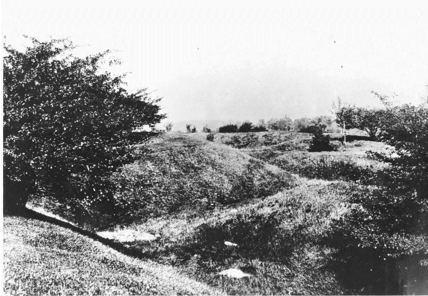
Figure 85 View of entrenchments at Old Fort Erie, undated photograph on file at Old Fort Erie, NHS.
