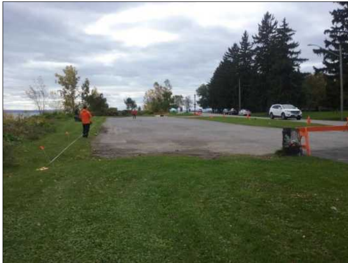
Figure 13. View of the parking lot looking south with baseline on east side.
