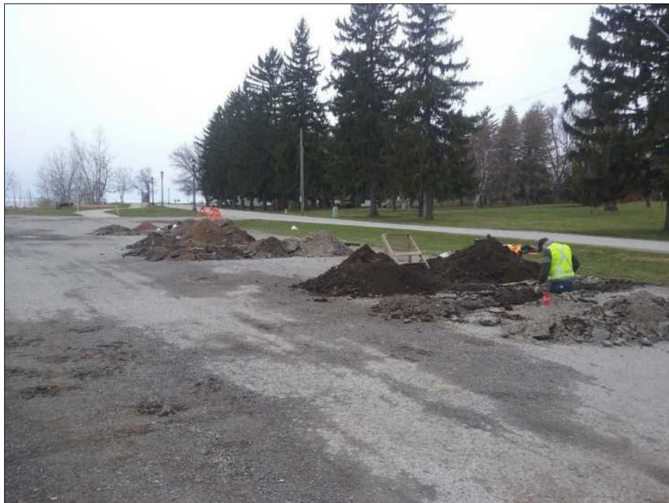
Figure 20. View looking south and west showing three trenches excavated on April 16 to verify GPR survey results of October 30, 2018. Trench 1 is in foreground and Trench 2 in background. Trench 3, is visible in the middle ground.
