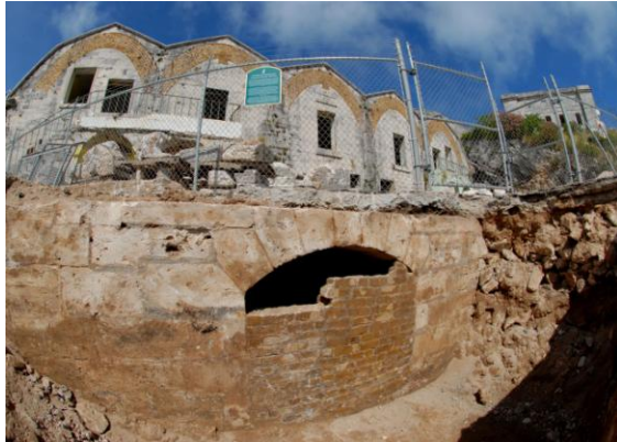
Figure 1 View of the blocked tunnel entrance, north end, shortly after discovery in June 2009. The bricks were removed to gain access to the tunnel which runs below the Lower Ordnance building.
