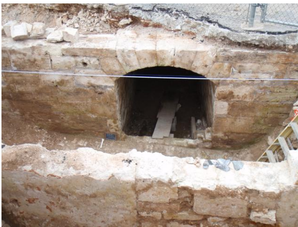
Figure 6 Photo of north terminus and wall, Phase I, with Stable/Store building in foreground (Phase III) and blocked doorway to right (Phase IV).
