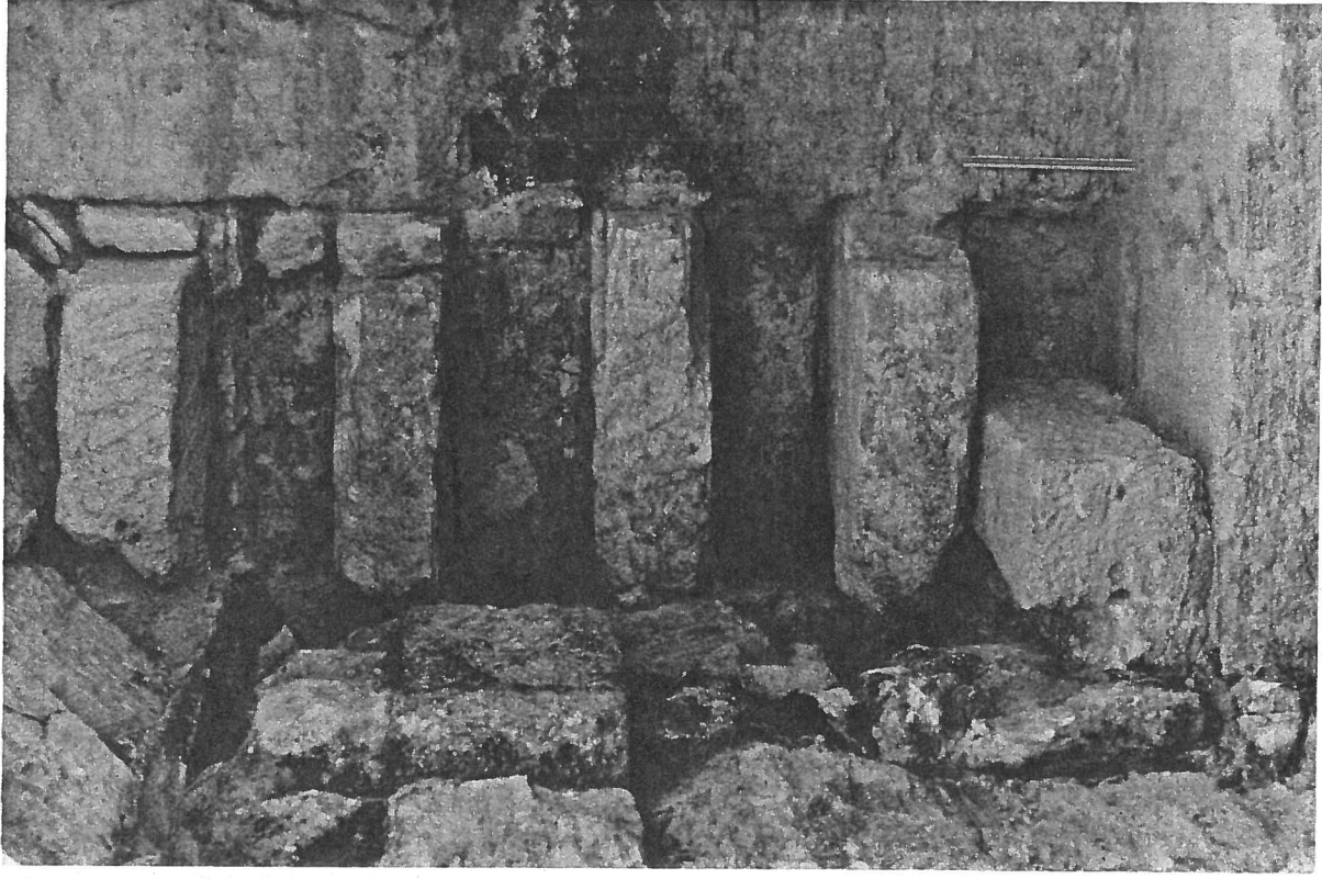
FIG. 11: Behind the inner blocking wall in Arch 20, the bedrock face contained an additional blocking of massive stones on the southern side of the Arch.
