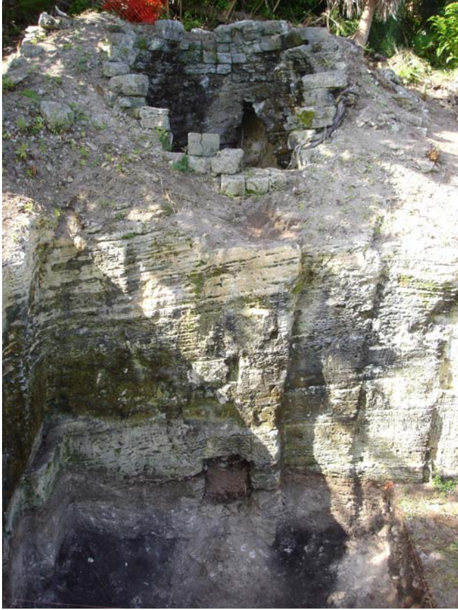
Figure 3 Lime kiln after excavation completed showing original surface of blackened bedrock opposite draw hole on bottom, quarry face, partially collapsed stack and charge hole at top.
