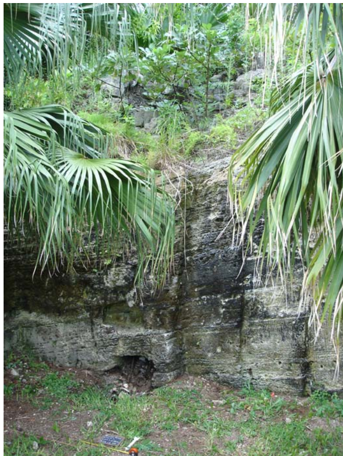
Figure 2 Lime kiln prior to clearing for excavation. Unit A opposite the draw hole is visible on quarry face.
