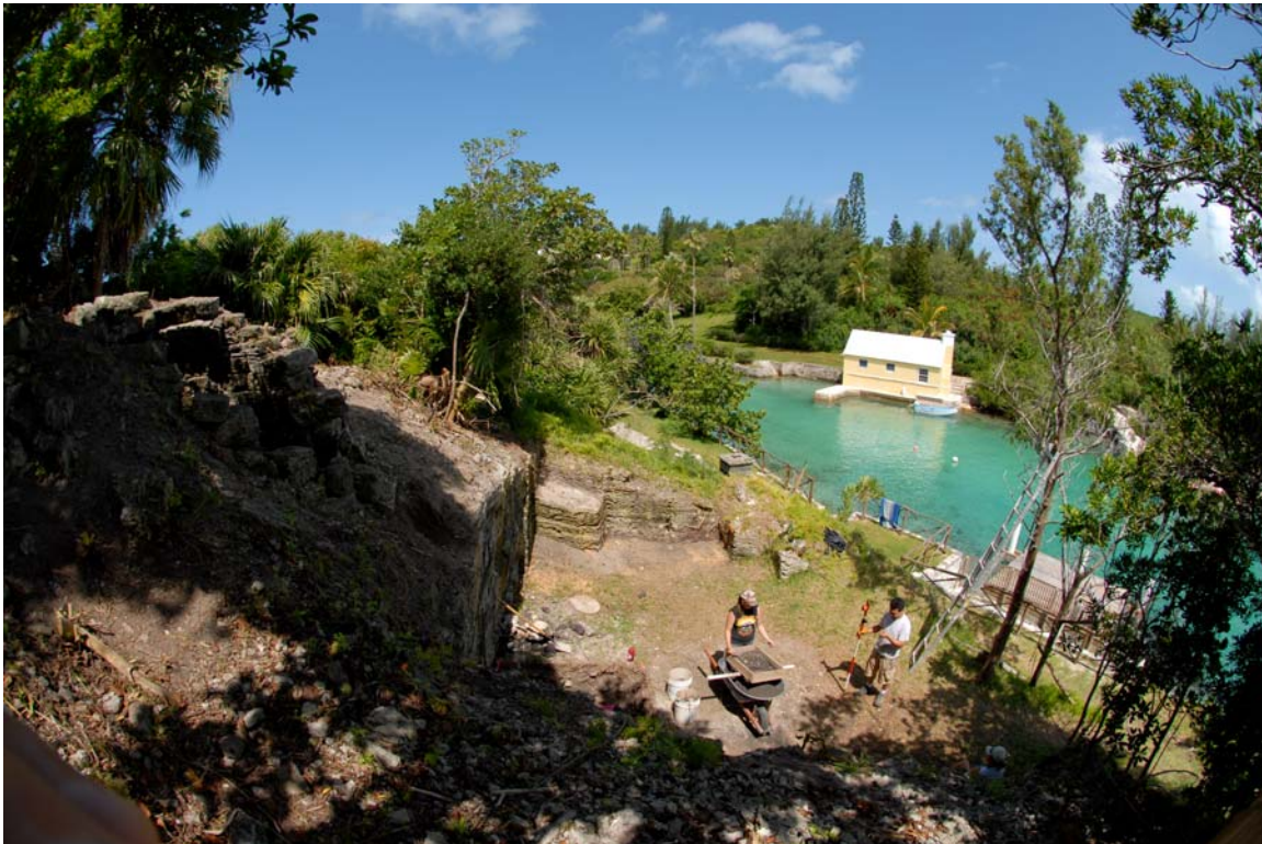
Figure 1 Teuser Place lime kiln on Scroggins Bay, Sandys. Lime kiln charging stack on left and quarried area below.
