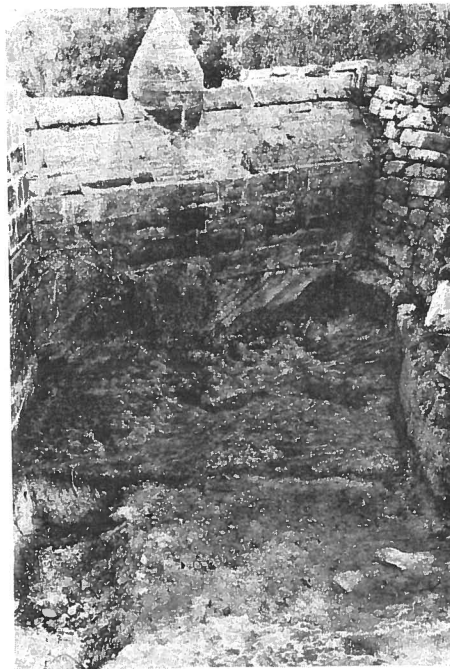
FIG. 5: View of the tapered breach in counterscarp revetment adjacent to batardeau.
